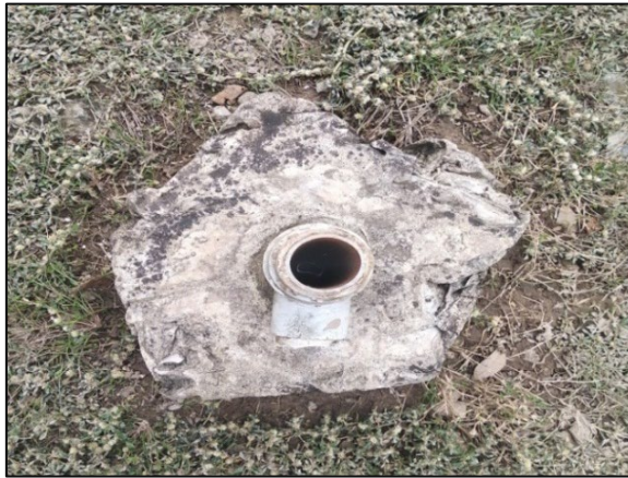
Fig. 4. Well no longer in use, but not yet safely sealed
