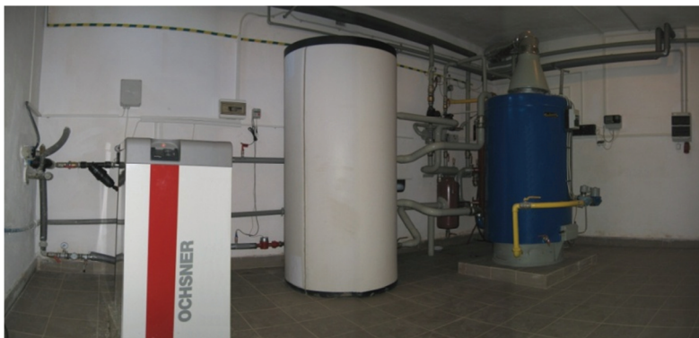
Fig. 4. Assembled heating system, heat pump, buffer tank, electricity distribution, water installation [1, 6]
