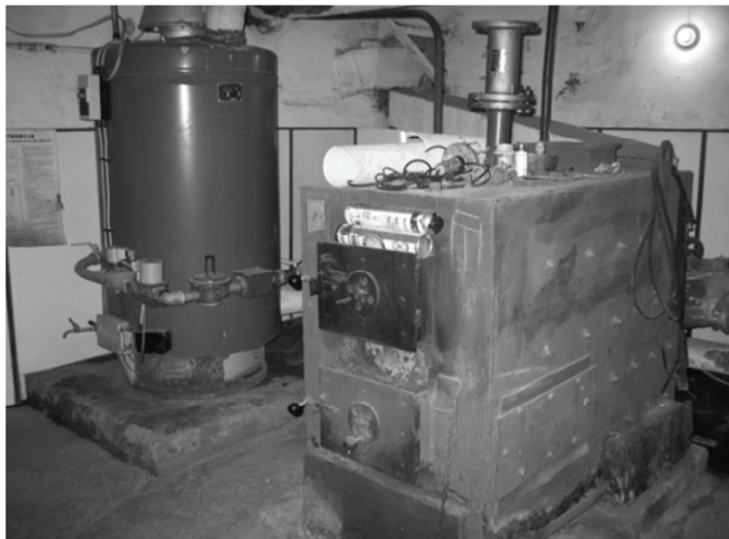
Fig. 2. Boiler room in school; Jubam gas boiler and an old coal boiler [1]
