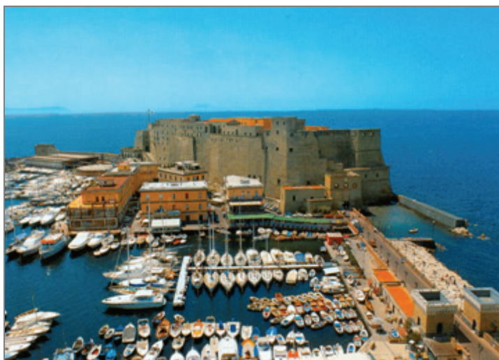
Fig. 1. The front part of Castel dell'Ovo in Napoli was constructed from tuffo napolitano
